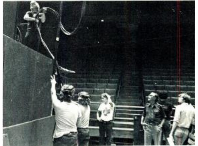
Claire Brothers P.A. Company technicians cabling their main speaker system.
