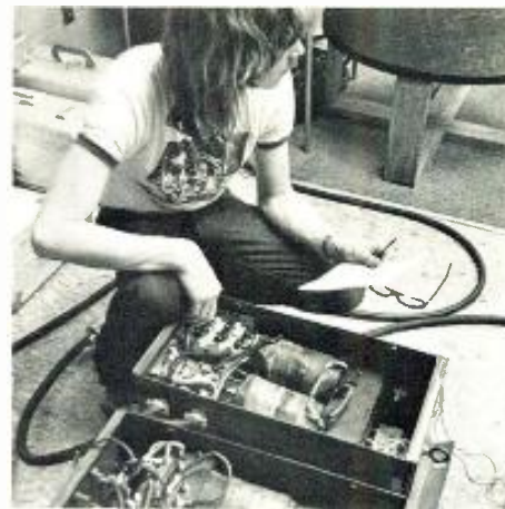
220-volt stepdown transformers being tapped for the optimum voltage.
